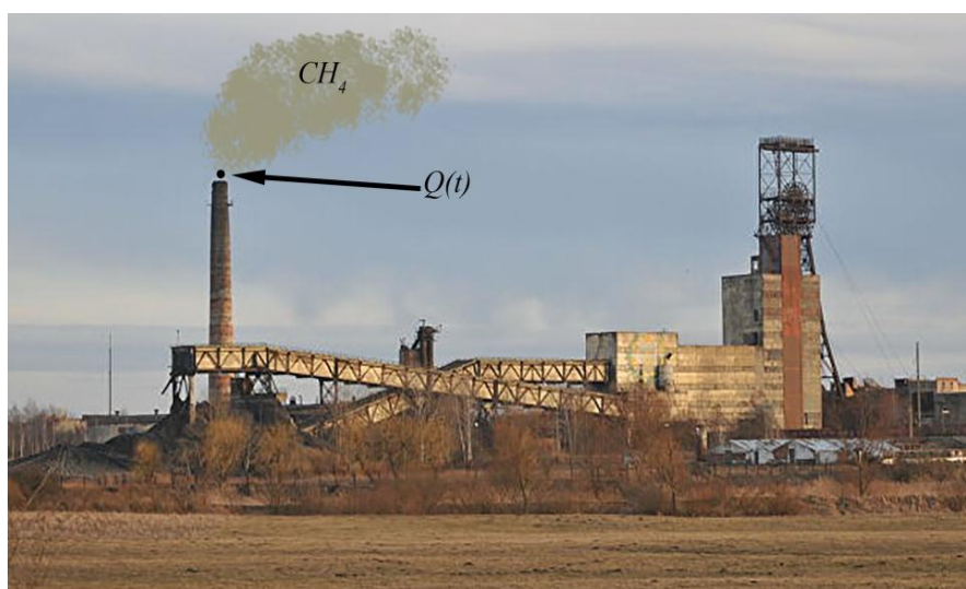
Figure 2 – Methane emission from the pipe
